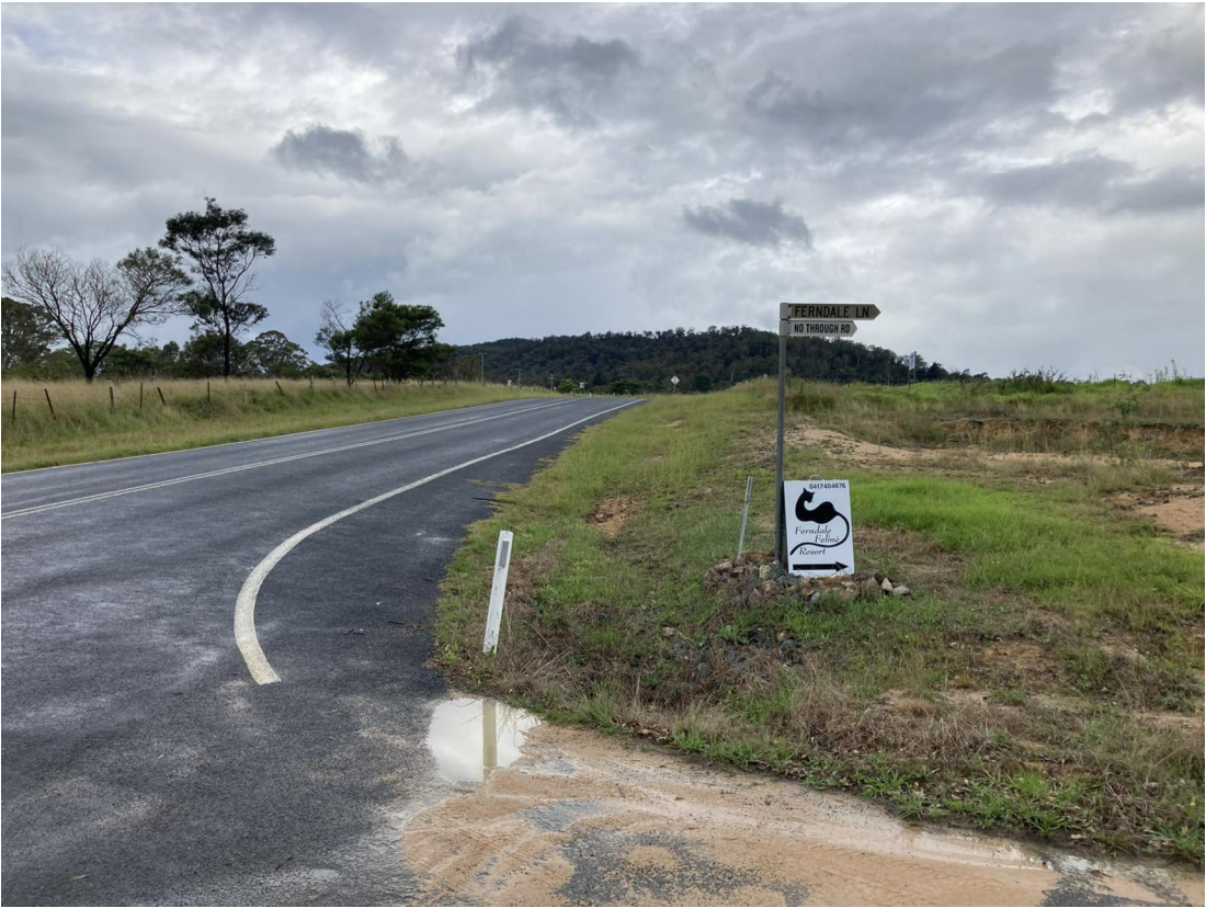
VIEW TO EAST FERNDALE LN > CANDELO WOLUMLA RD
